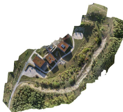
Fig. 1. Drone model of Rzepka Quarry, rehabilitated in a recreational area, mapped using DJI Phantom 4 on 30.09.2018. Field work of approximately 5 minutes and 1 hour of data processing
