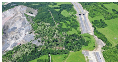
Fig. 7. The 2013 landslide at its largest extent. The thin silvery line represents the damaged and still non-functional railway line [20]
