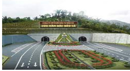
Fig. 2. Deo Ca traffic tunnel
