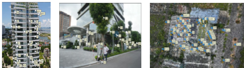
Fig. 11. Distribution of image control points and checkpoints for high building
