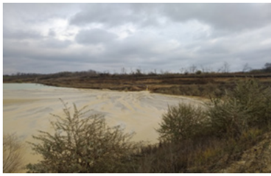
Fig. 2. Concentrated release of tails from the pulp duct Rys. 2. Skoncentrowane uwalnianie odpadów
