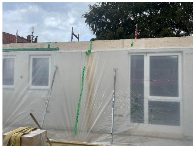
Fig. 1. Carefully protected element before ceiling is assembled in hybrid construction
