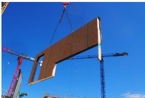
Figure 2. Wall section transferred by crane without pre-installed protection
