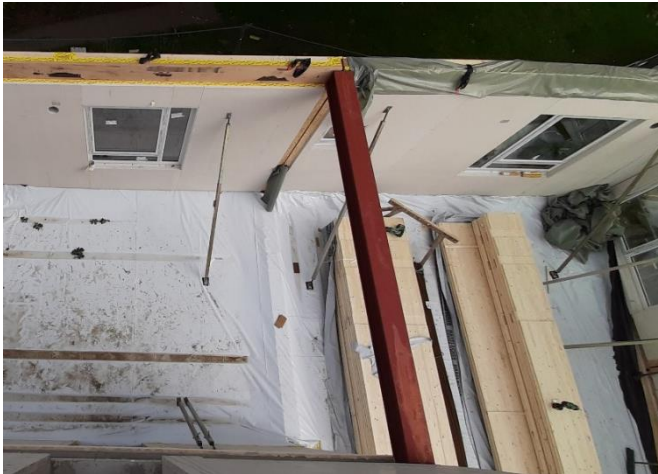
Fig. 4. Ceiling elements and upper wall sections covered with foil
