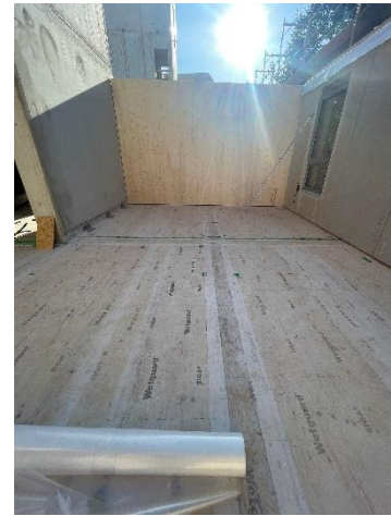
Fig. 5. Ceiling protected by fully bonded translucent membrane
