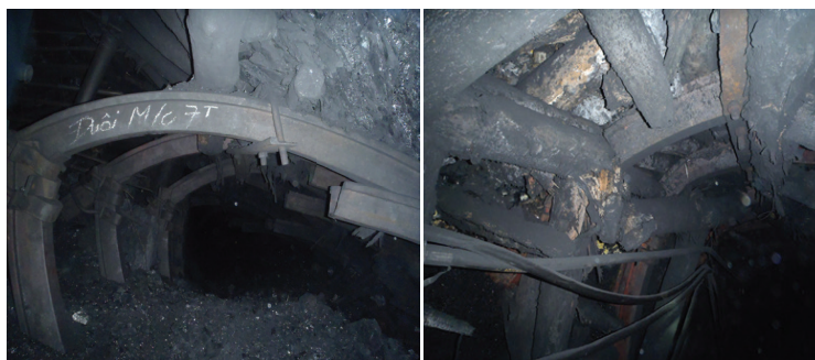
Fig. 5. The collapses of drift at seam 10 level -25 in Mao Khe coal mine, Quang Ninh province [2]
