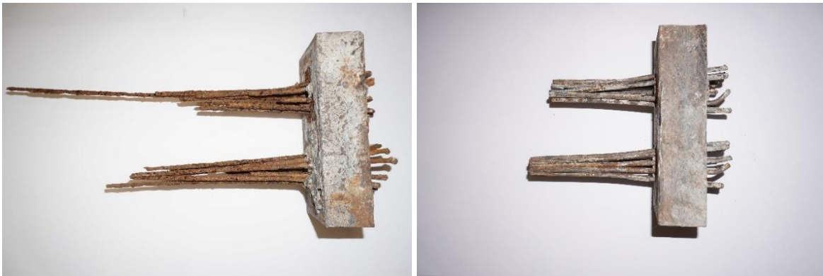
Fig. 13. The upper anchor in the location of the truss bedding on the column – – total corrosion of the tendons and opposite side in the relative satisfying condition – taken out from the collapsed truss
