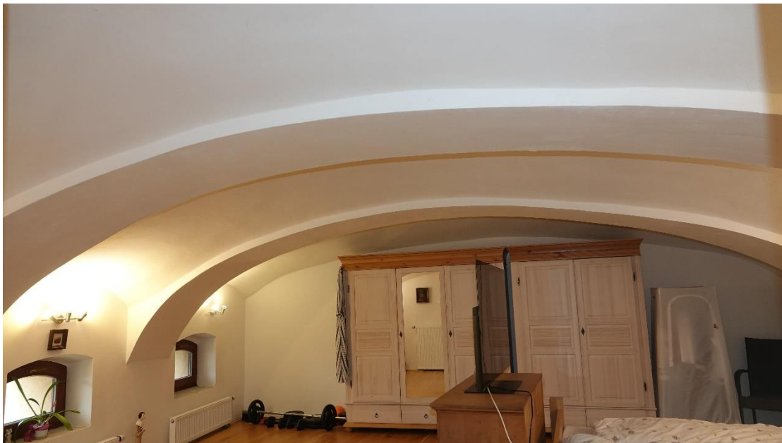
Fig. 9. Today's view of the space under the prestressed arches
