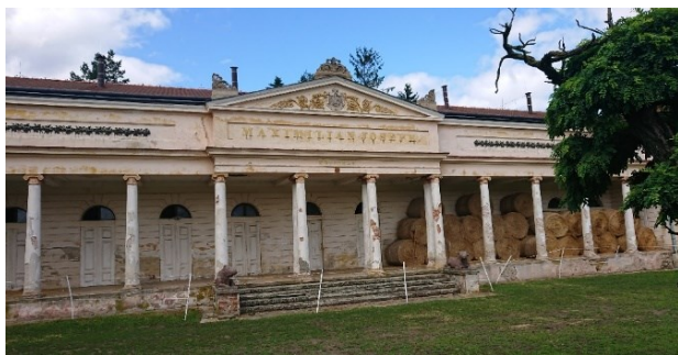
Fig. 1a. Hubertcentrum building
