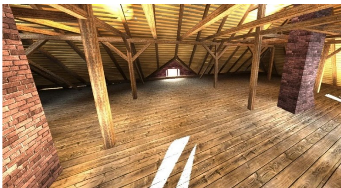
Fig. 2a. View of the roof of a building in Cetkovice
