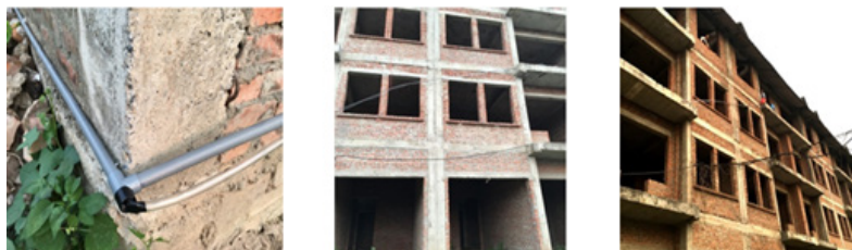
Fig. 6. The area for the experiment of backfill materials transportation
