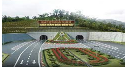
Fig. 2. Deo Ca traffic tunnel
