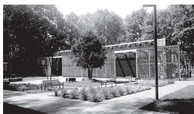
Fig. 5. Saline graduation tower in Katowice (K. Tobór-Osadnik's foto)
