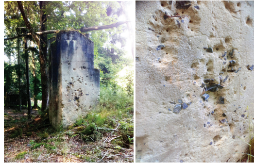
Fig. 6. The pillar of former stone crusher and its detail Rys. 6. Fundament dawnej kruszarki kamienia i jego detal
